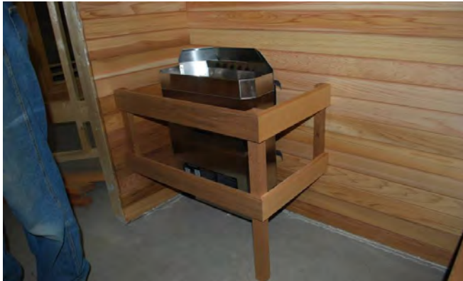
140. Place heater guard into place.
