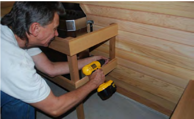
151. Screw opposite side into wall.
