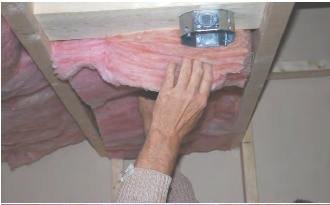
56. Fitting insulation around light.
