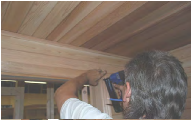
177. Measure from floor to top casing and cut side casing to fit. Attach with finishing nails
