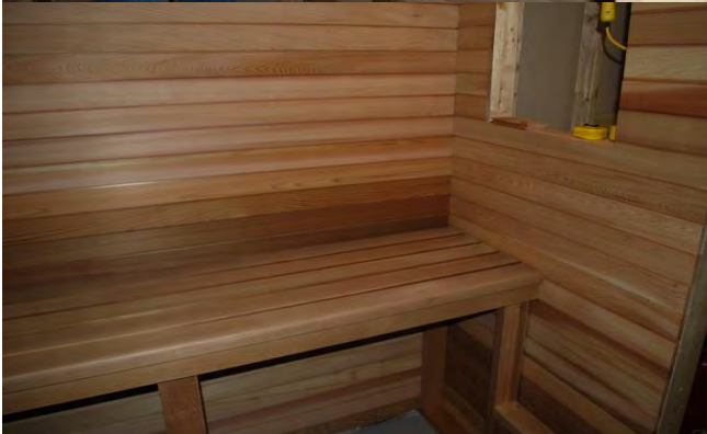
112. Flip up top bench and faster frames to wall.
