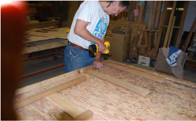
129. Screw 15" vertical onto 1x4 horizontal.
