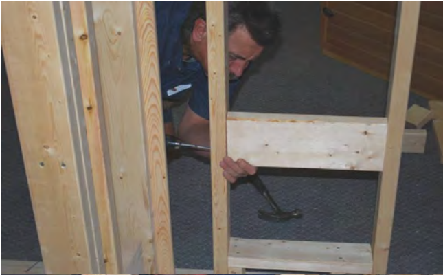
36. Installing backing for bench hangers.
