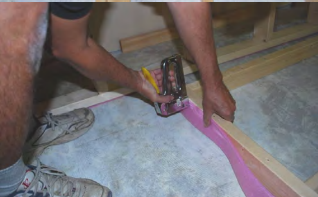
15. Staple sill gasket to bottom plate to prevent moisture from coming into contact with wood. Pressure treated wood should never be used indoors.
