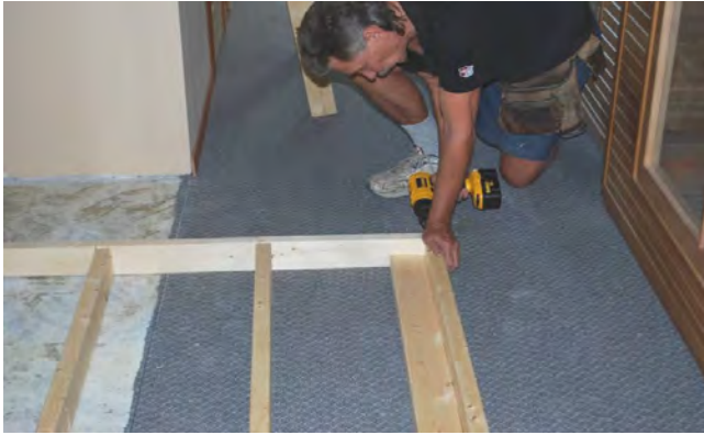
13. Screw or nail L-frame to bottom plate.
