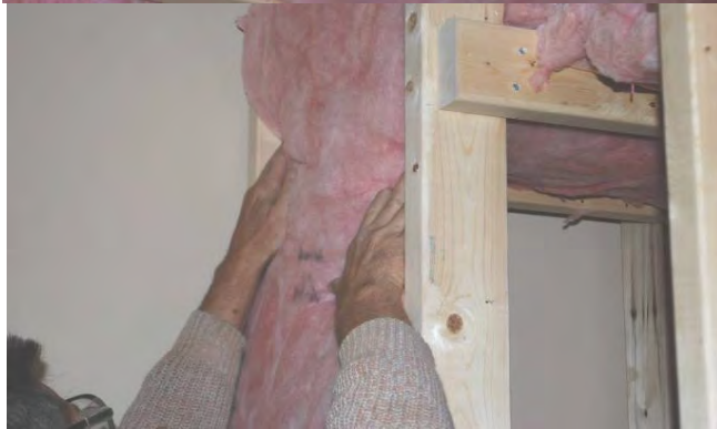
58. Use minimum of R-12 in walls. Make sure insulation is for 16" O.C's. Fit insulation between wall studs.
