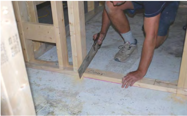
40. Cut out base plate between door studs.
