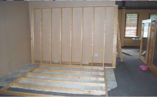
16. Lay up adjoining wall. Screw together and staple gasket to bottom plate. (The side walls will not have the L-frames)
