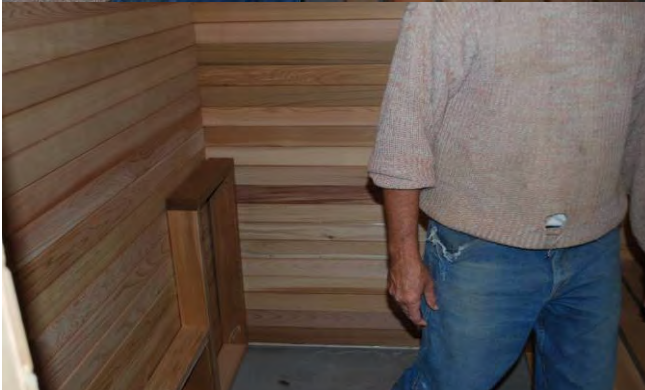
121. Secure frame to wall in corner.
