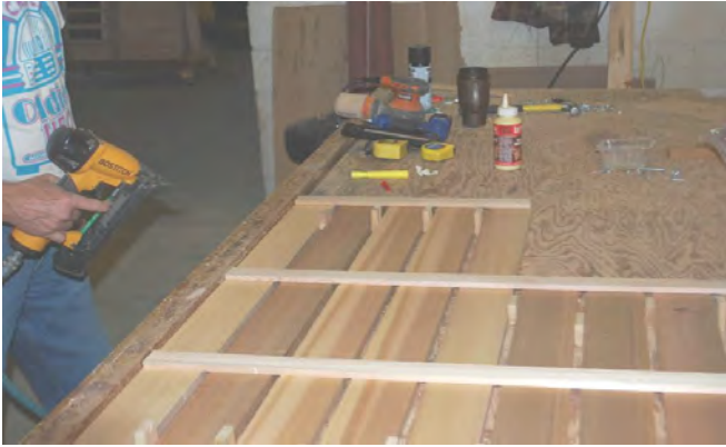
157. Depending on the shape and size of floor will determine number of sleepers.
