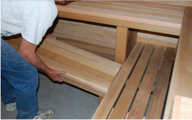
124. Bench that sits on frame, only the fascia needs to be installed past the bench top.
