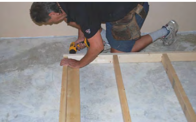
14. Screw studs into place. Picture shows screwing opposite L-frame into place.
