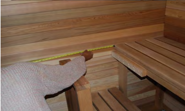
122. Measure from bench top to corner. Subtract \frac{1}{4} " to fit.
