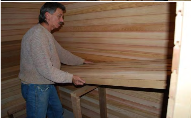
111. Top bench in place. Make sure center bench frame is lined up with center x-pc.
