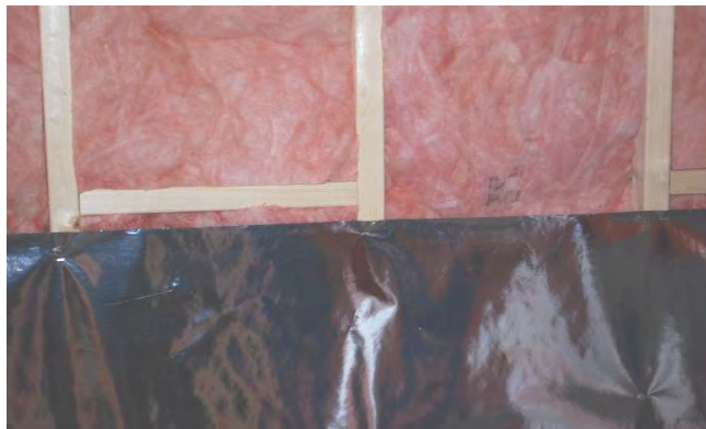
59. Installing the foil vapour barrier: Start at bottom and roll foil vapour barrier out. Staple to studs at the top, bottom and centre. The shiny side faces into the sauna.
