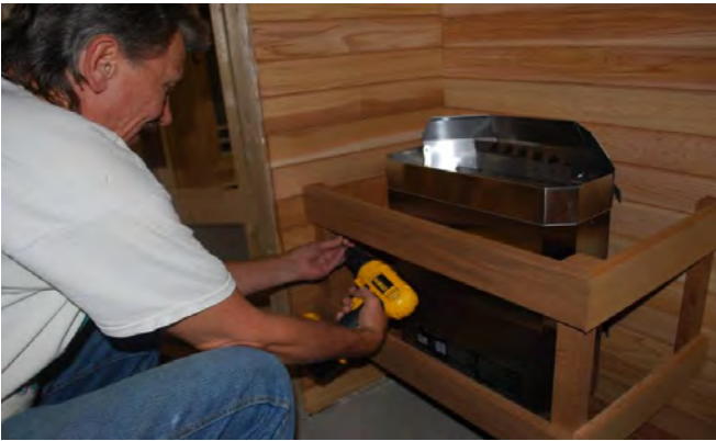
150. Screw heater guard into place through 15" pieces.
