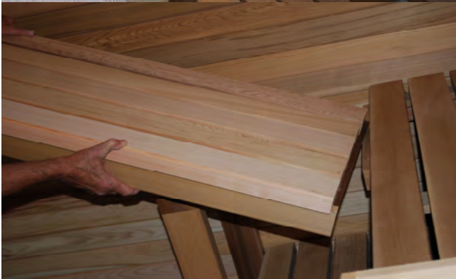
123. For L-benches that will sit on a bench hanger cut fascia \frac{1}{2} " longer than bench tops. Install fascia and cross piece, \frac{1}{2} " past bench tops on end of bench that sits on hanger. Make sure cross piece will line up with bench frames.
