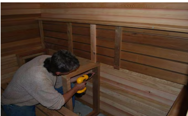
113. Place bottom bench into position on top of frames.
