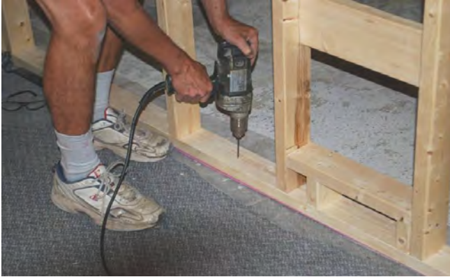
38. Drill holes to attach base plate to floor.
