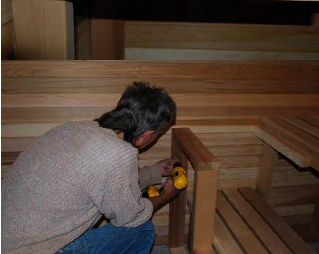
120. Secure bench frame to wall flush to bottom bench.
