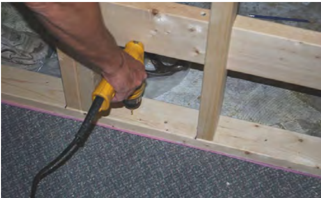
39. Use tap cons to secure base plate.
